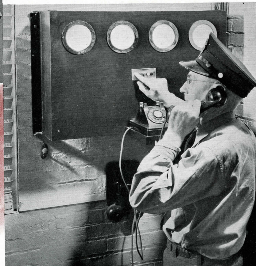
The Air Raid Warning System (right), and the Plant Blackout Control System (above), are ready to function instantly. Warnings that come in to the Area Control Center are relayed promptly to the "Caterpillar" Control Board. The distance of approaching planes, in terms of minutes, is indicated by one of four colors on the Control Board. The officer on duty has only to punch a button to set off the plant warning system. At once, the Blackout System functions, with trained men, near each of 30 locations, rushing to pull the switches and disconnect all sources of artificial light.
